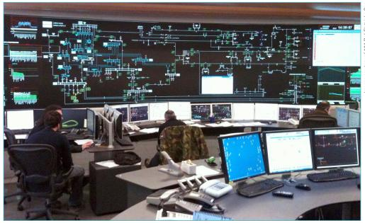
A2A uses 19 Matrox Extio Series KVM extenders to remotely drive 19 multi-display operator stations in their new control room center.
