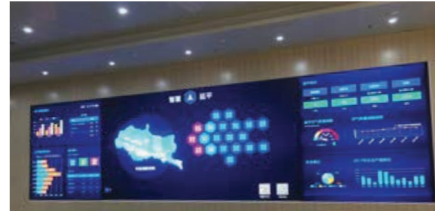
Telecom Bureau, Nanping
